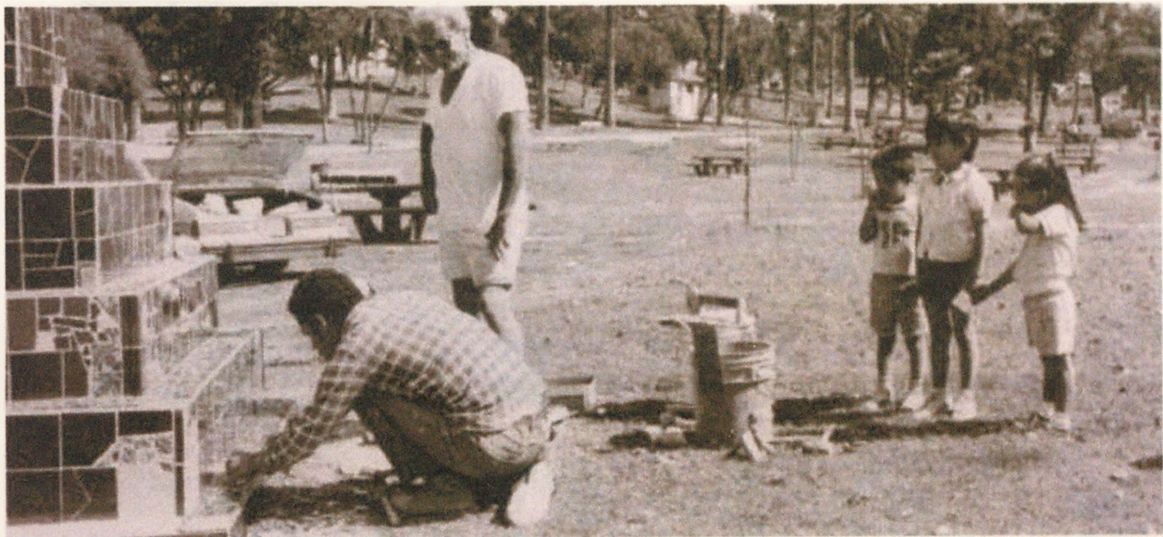
Installing ceramic tile covered pyramids in presence of community onlookers.
